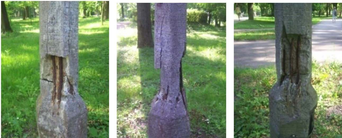
Figure 1: Damage of the lighting pole.
