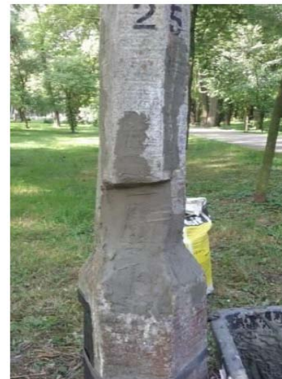
Figure 2: Application of the mortar contact layer Ceresit CD 30.
