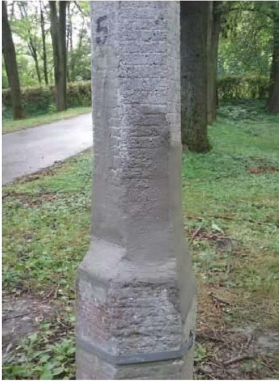
Figure 3: Application of finishing layer with mortar Ceresit CD 26.
