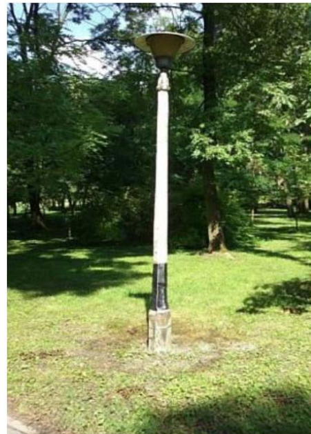
Figure 5: The final effect of the lightning pole repair.
